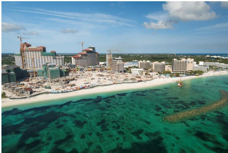
**Figure 3: Submerged breakwater and sand nourishment on the new Bahamar beach in The Bahamas**
